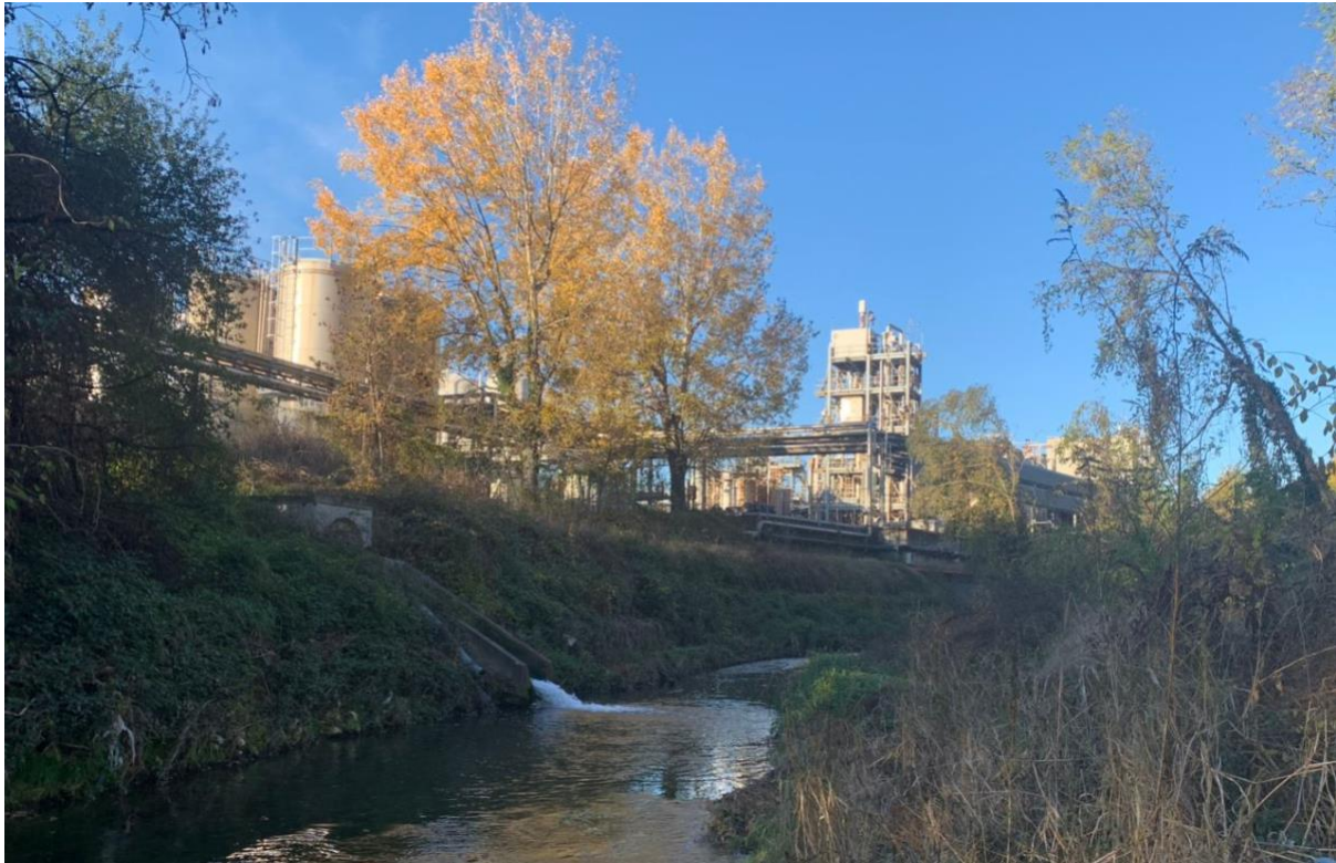
Figure 6: A drainage canal that discharges into the Poscola stream behind the Rimar-Miteni plant in Trissino, Vicenza (photo by the author, January 2020).
